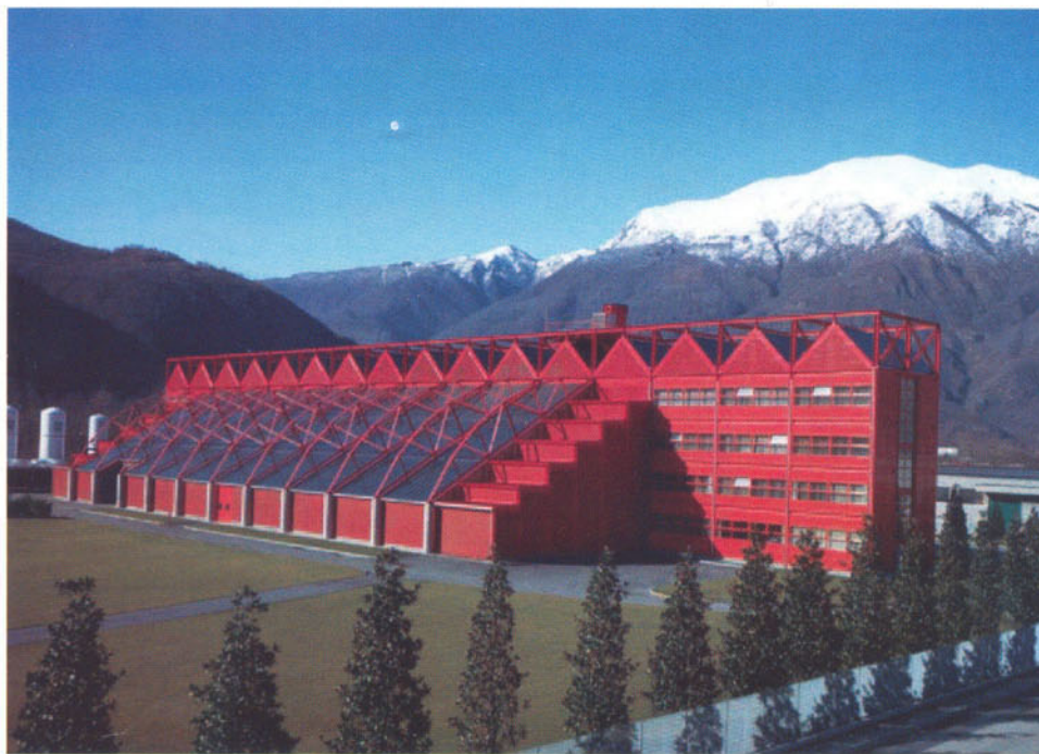
The demonstration plant in operation during 1992–1998 at Fondotoce, Italy, accepted MSW and industrial wastes, and used the resulting syngas for electricity production
